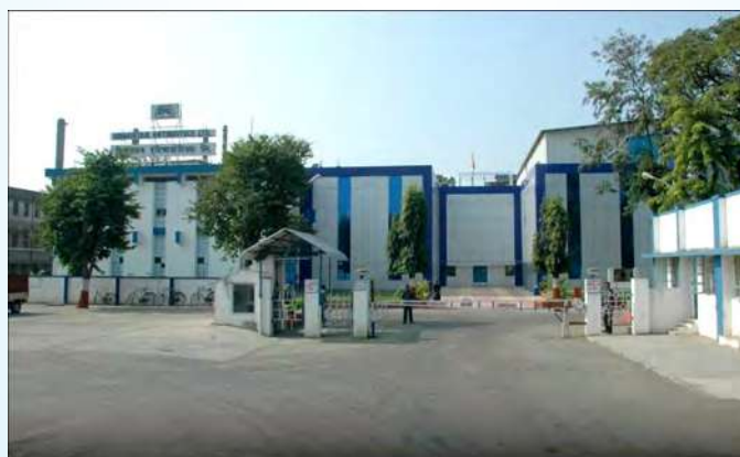
HAL - Building Front View Of Cephalosporin Plant
